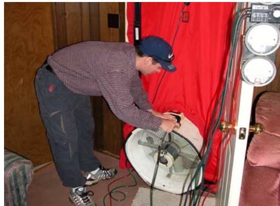
Before & after blower door tests quantify energy savings
